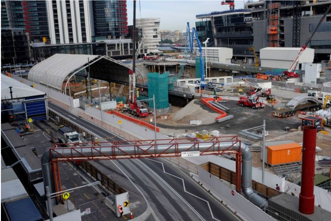
Figure 7. Hickson Road cut through the site of the gasworks and now provides a dividing line for the Western side of the site (right), which was decontaminated by late 2018, and the Eastern side (left), which is still undergoing remediation. Image courtesy of the author.
